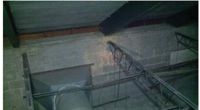
Photograph 4 – This photograph illustrates the bearing condition at the eve of the Campus Center building.
