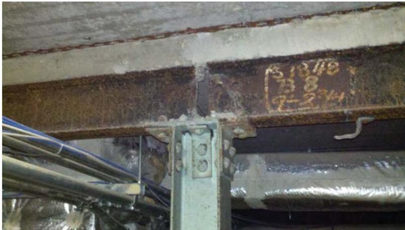
Photograph 3 Photograph 3 illustrates the corroded condition of the structural steel that supports the floor system in the central portion of the building.
