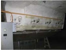
Access to mechanical units is difficult throughout Trinkle Hall. In many cases, a small access panel is the only way to get to a unit. In addition, the units are often located in congested areas making maintenance a further difficulty.
