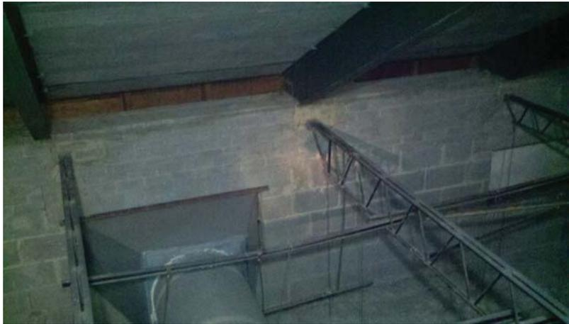
Photograph 4 – This photograph illustrates the bearing condition at the eve of the Campus Center building.
