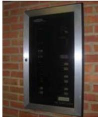
The Fire Alarm Control Panel is an older Faraday 7800 panel that will be difficult to upgrade to maintain code compliance. The zone of the alarmed device is indicated at the control panel, with no distinction between the types of devices that are in alarm. For example, all of the kitchen hood alarms are on a single zone. This is in contrast to a more modern addressable system, in which each initiating device is individual monitored by the system.
