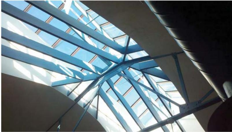
Photograph 2 – Roof framing in the central atrium of Trinkle Hall. In this photograph the primary roof supporting element is a steel truss, while the secondary framing consists of wood joists.
