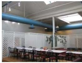
The air distribution throughout the Campus Center Building has increased comfort and efficiency, with several multi-zone air-handling units located within the attic. Each air-handling unit is provided with low-pressure steam for heating and chilled water for cooling. Zone dampers are located downstream of the unit and provide independent “turn-down” of the airflow to each thermostatic zone. Several units also contain hot water reheat, providing a better level of comfort control.
